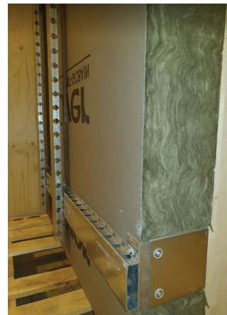
Fig. 10 SerpoVent U Wall bracket parts A-B, and SerpoVent hat sections installed in OL-33 insulation and CLT board
